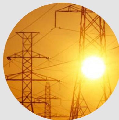
Electrical power supply
